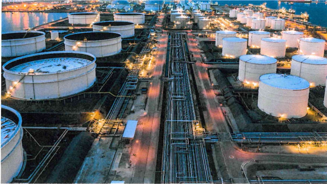
Figure 26: Kampala Storage Terminal
